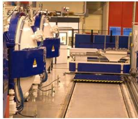
Vacuum Furnace Installation
