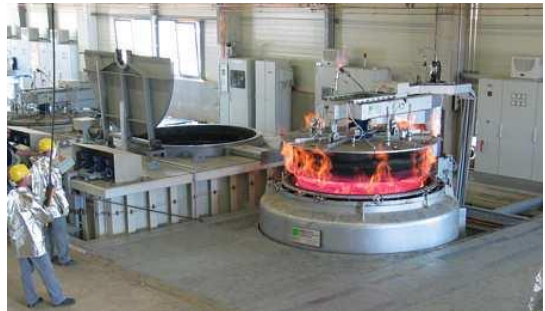
Figure 1: Pit Furnace Installation
